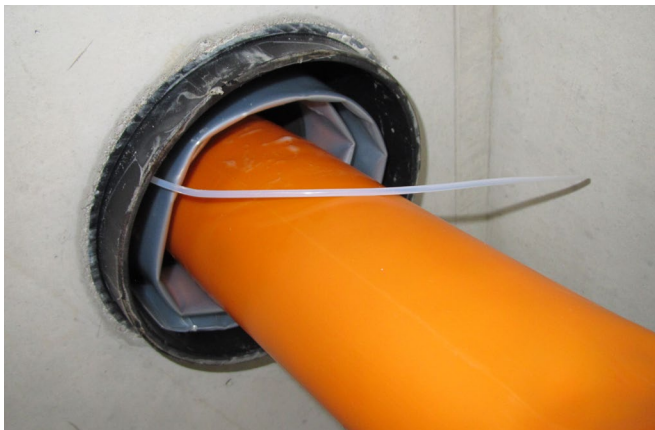
Combined installation of the TE connectivity ADE / TDUX in the KKR 110.
