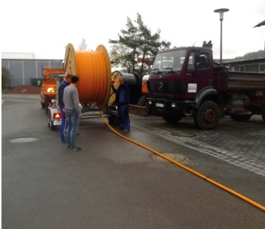
Unwinding SRV-G tc from the coil
