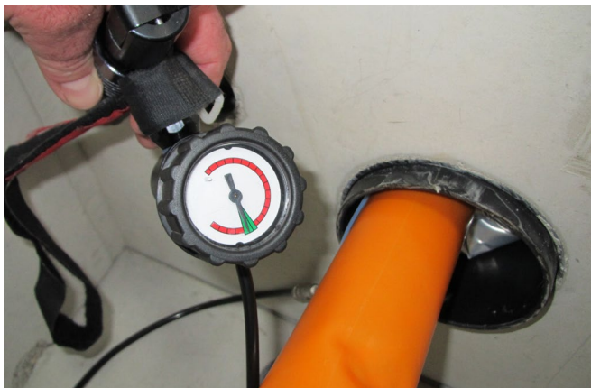
Filling and sealing the TE connectivity ADE / TDUX.
